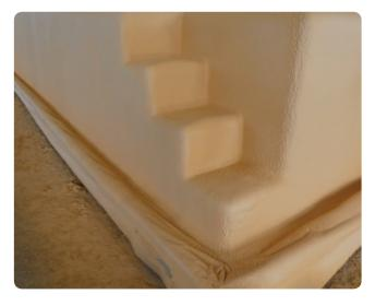
Foam insulation is applied to your swimming pool ensuring the water temperature is maintained at a higher temperature for longer than a non-insulated pool. This means better heating efficiencies and less ongoing cost in heating your pool.
