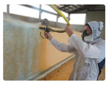
An outer skin of hard fibreglass adds further structural strength to your Bermuda pool and protects the polyurethane insulation.
